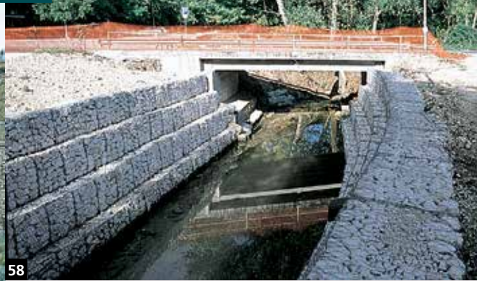
58. Hydraulic protection with Terramesh® S and gabions, Vella river, Sulmona (AQ)-Italy.
