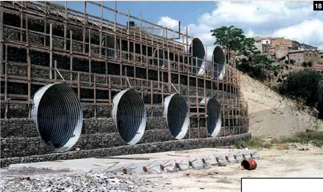
18-19. Road embankment in Terramesh® S and geogrids, Aliano (MT)-Italy.
