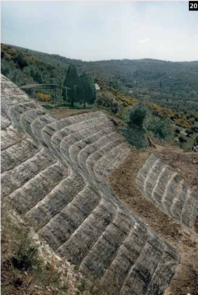
20-21. Slope stabilization in geogrids, Passignano (PG)-Italy.
