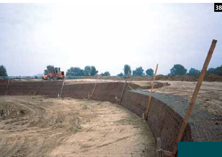
38-39. Green Terramesh® retaining wall, Civitanova Marche (MC)-Italy.
