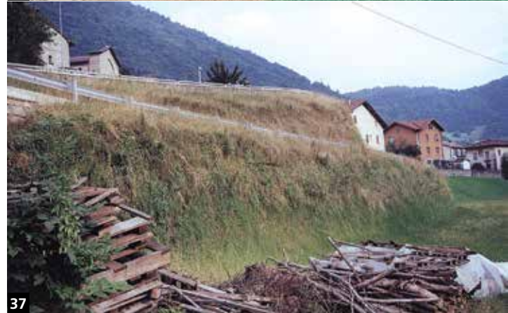
35-36-37. Road restructuring using Green Terramesh®, Valle d'Ogna (BG)-Italy.
