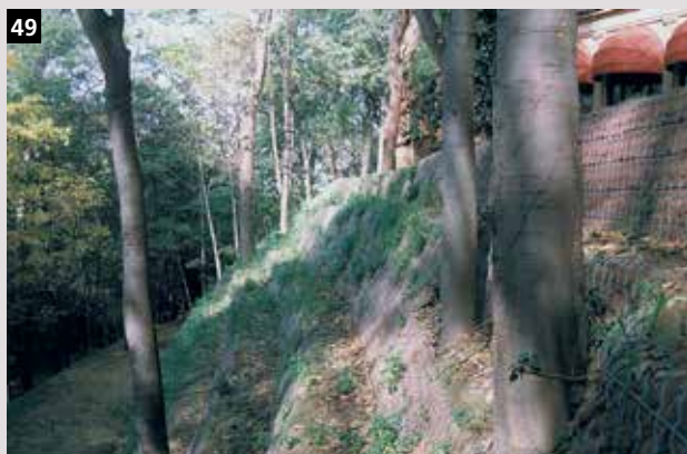
49. Green Terramesh® retaining structure, Bologna-Italy.
