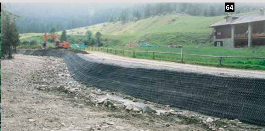
64. River bank protection with Green Terramesh® Water, Cogne (AO)-Italy.
