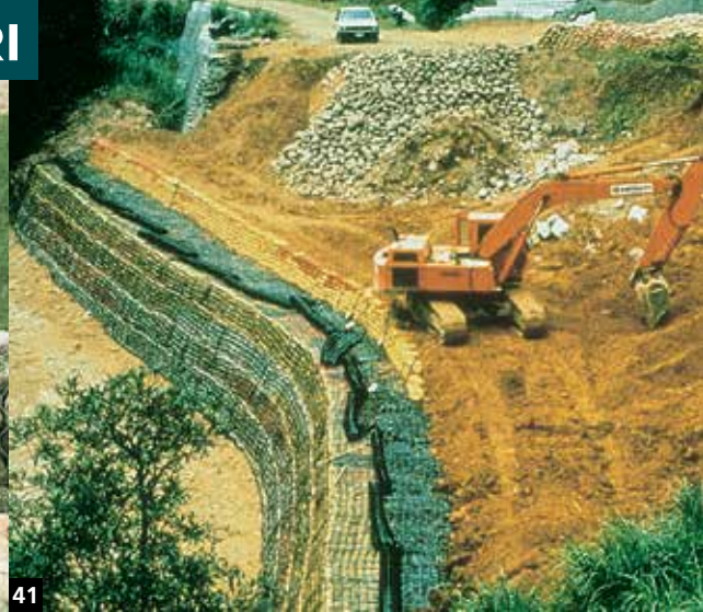
40-41. Slope stabilization with geogrids, Tapei-Taiwan.
