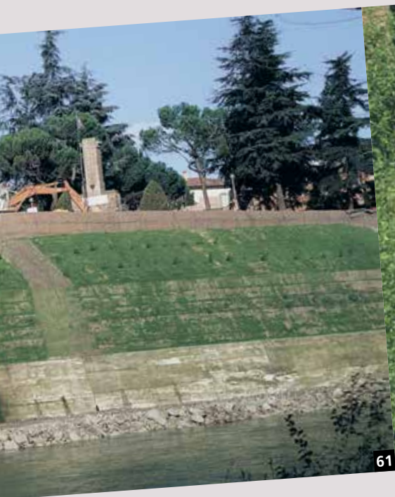
63. Geogrids retaining structure for enlargement of a road, Arcola (SP)-Italy.
