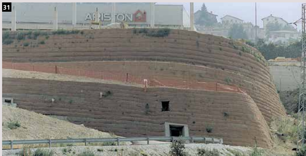
31, 32. Retaining structure in Green Terramesh® to extend industrial building, Arcevia (AN)-Italy.
