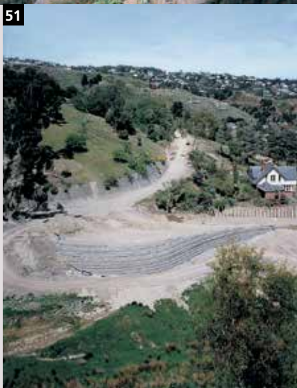
51. Retaining structure with Terramesh® S for new residential area, Christchurch, -New Zealand.
