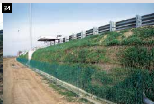
33-34. Green Terramesh® retaining structure to extend toll barrier, Villesse (GO)-Italy.
