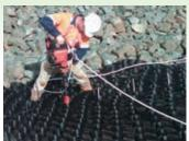
Presto's ATRA® anchors make a secure connection with the GEOWEB® cell wall and are fast and easy to drive with ATRA® drivers.
