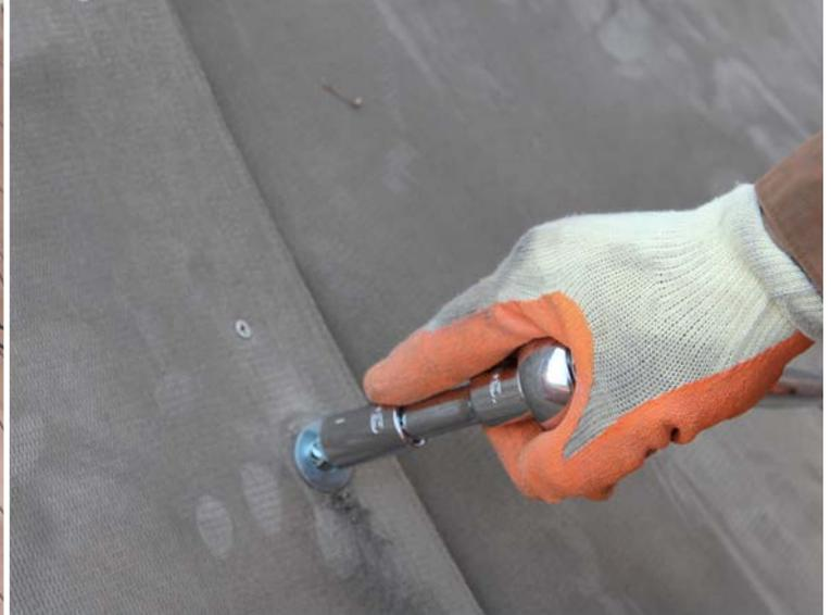
CC fixed to slope using rock bolt
