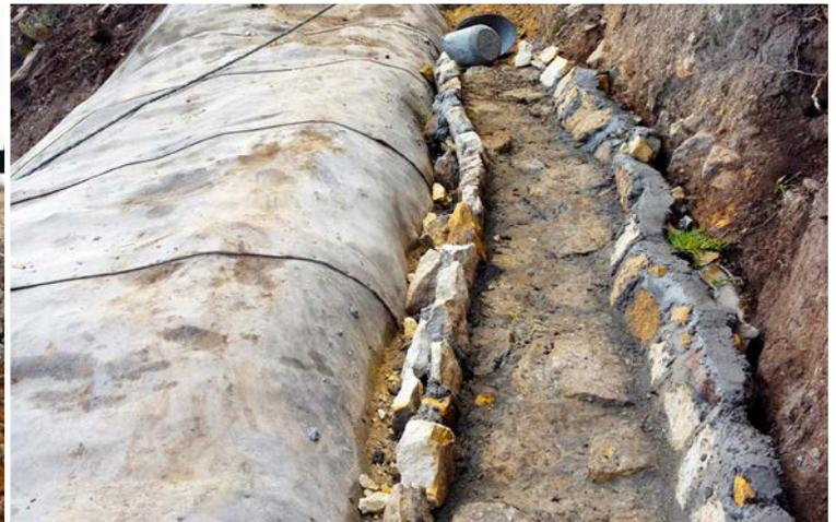
Concrete anchor trench constructed over CC at the crest of a slope
