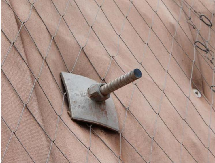
Rock bolt and large anchor plate with radiused corners
