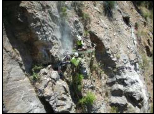
Figure 3. Drilling and installation of fence anchors
