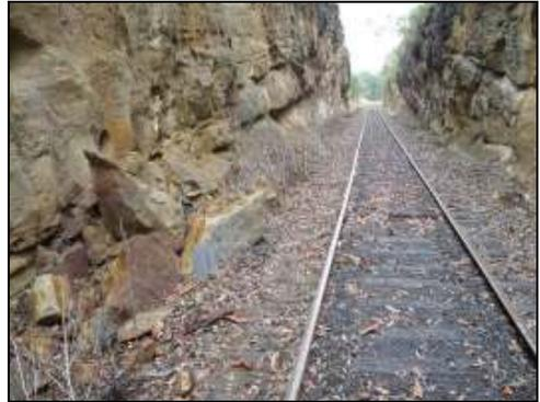
Figure 8. Rock falls near the railway line
