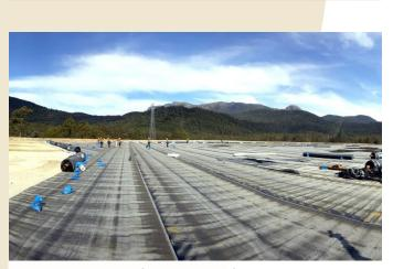
Teranap was chosen for this project for its weldability and flexibility to conform to irregular shapes and surface conditions.
