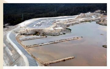
Geotas installed 190,000 m<sup>2</sup> net area of the Teranap 531 liner and 250,000 m<sup>2</sup> of upper and lower bidim cushioning geotextile.
