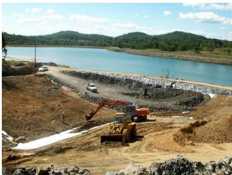
In order to recover precious metals from the flue dust material, an above-liner collection system was specified using a **Megaflo<sup>®</sup>** Flat Panel collection system.
