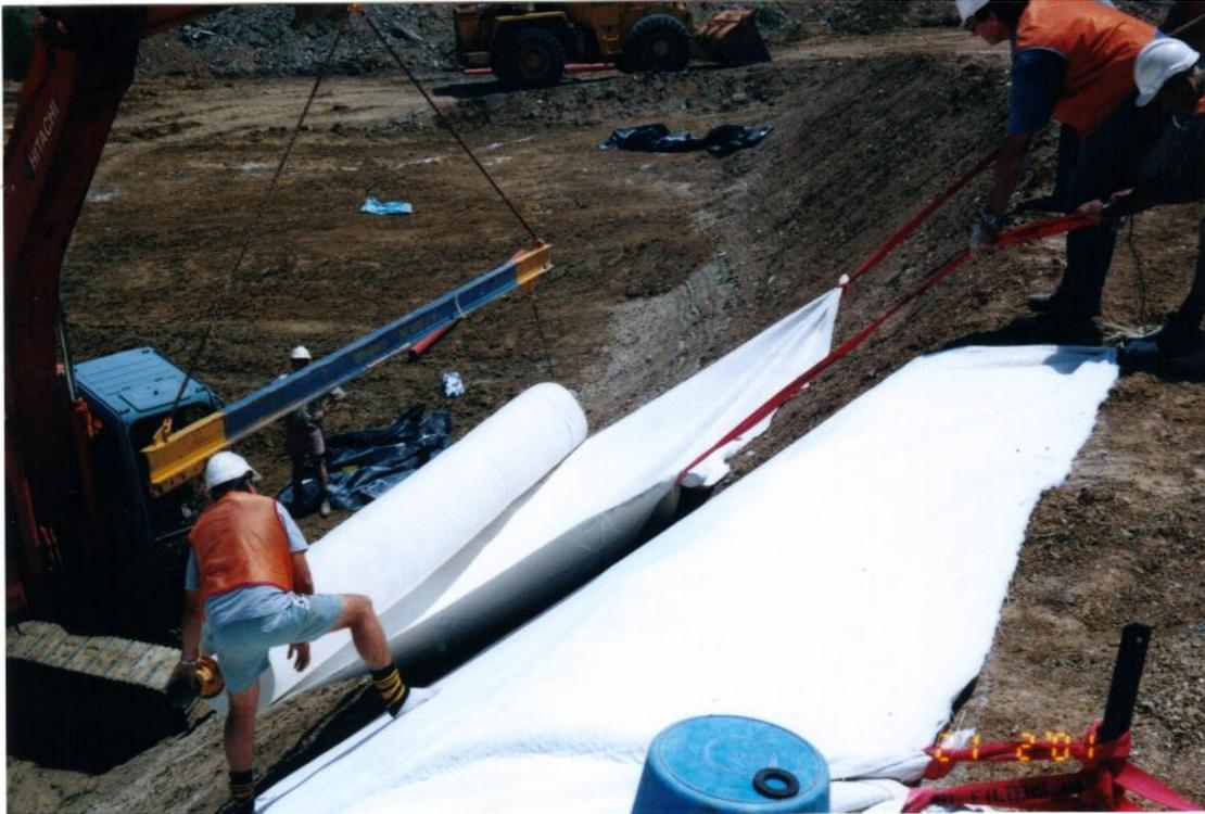
**Photo 1 – Installation of ELCOSEAL GCL on the upstream tailings dam face**
