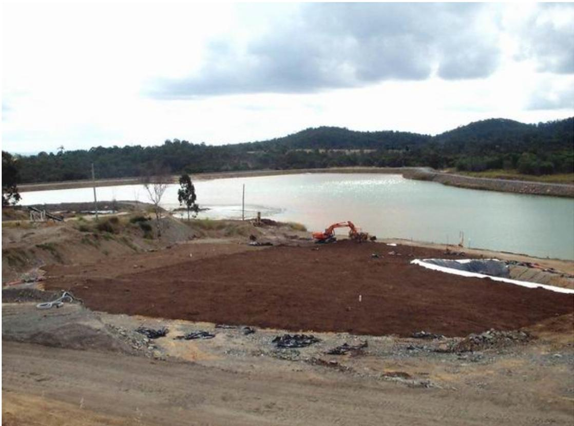
**Photo 6 – Completed cell with leachate dam on RHS**
