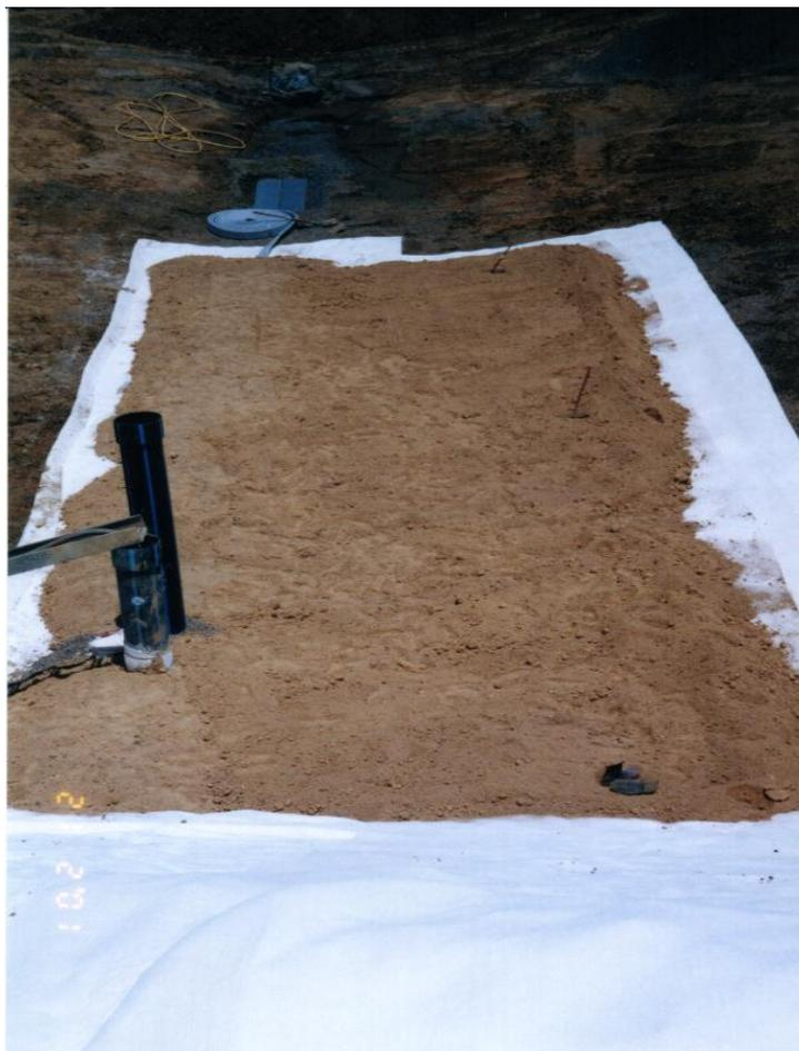
**Photo 2 – Placement of cushioning material on GCL**
