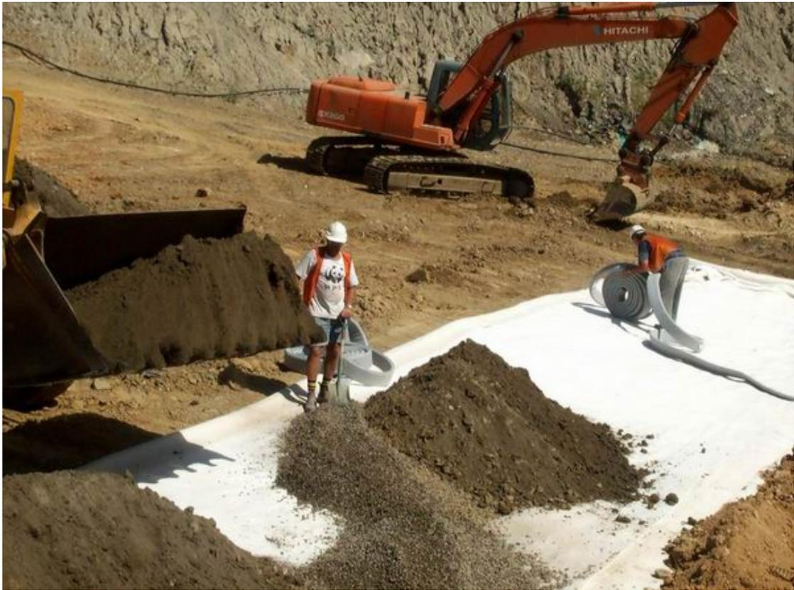
**Photo 3 – Installation of Megaflo over-drainage on GCL**
