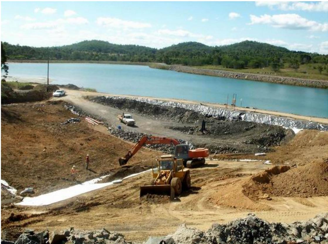
**Photo 4 – Placement of waste rock & cover material**
