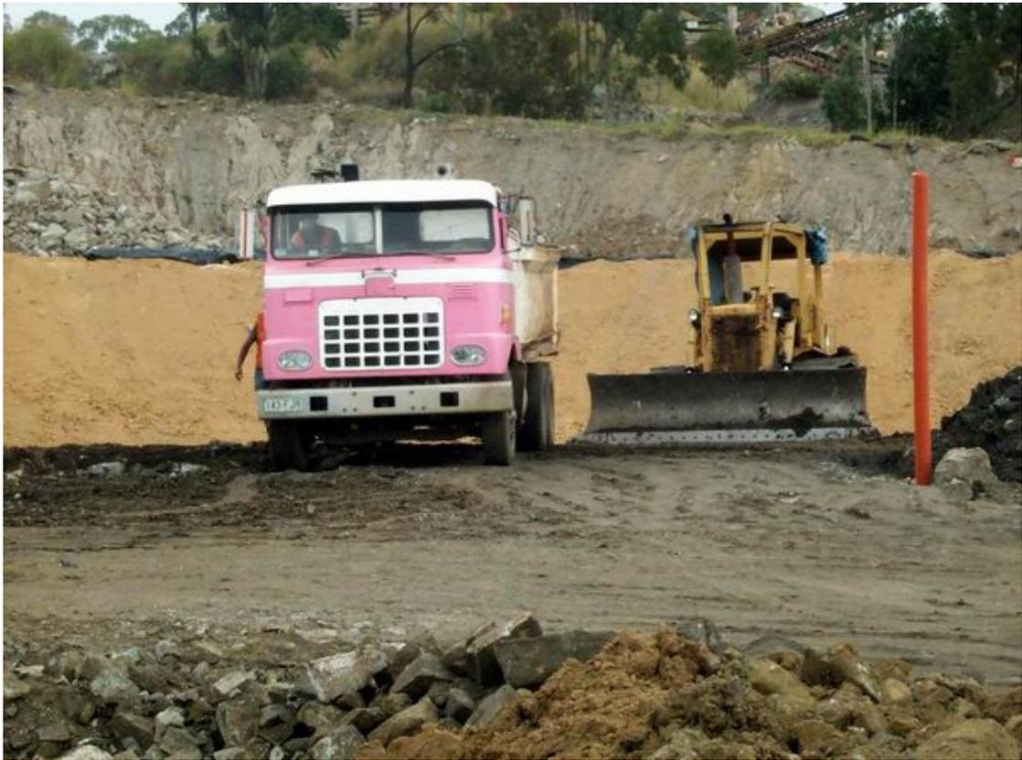
**Photo 5 – Filling of containment cell**
