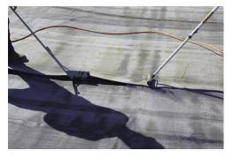
Aeramix technicians were properly trained to install the Teranap according to Siplast recommendations. Teranap was easily fully bonded directly to all concrete structures to make a watertight structural seal using Siplast primer and then torching. Ends were finished using termination bars.
